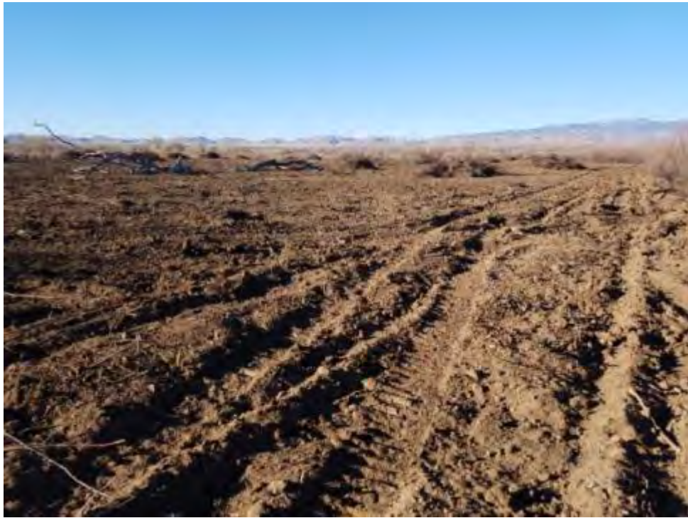
A large, completed area following root plowing in 2 directions.
