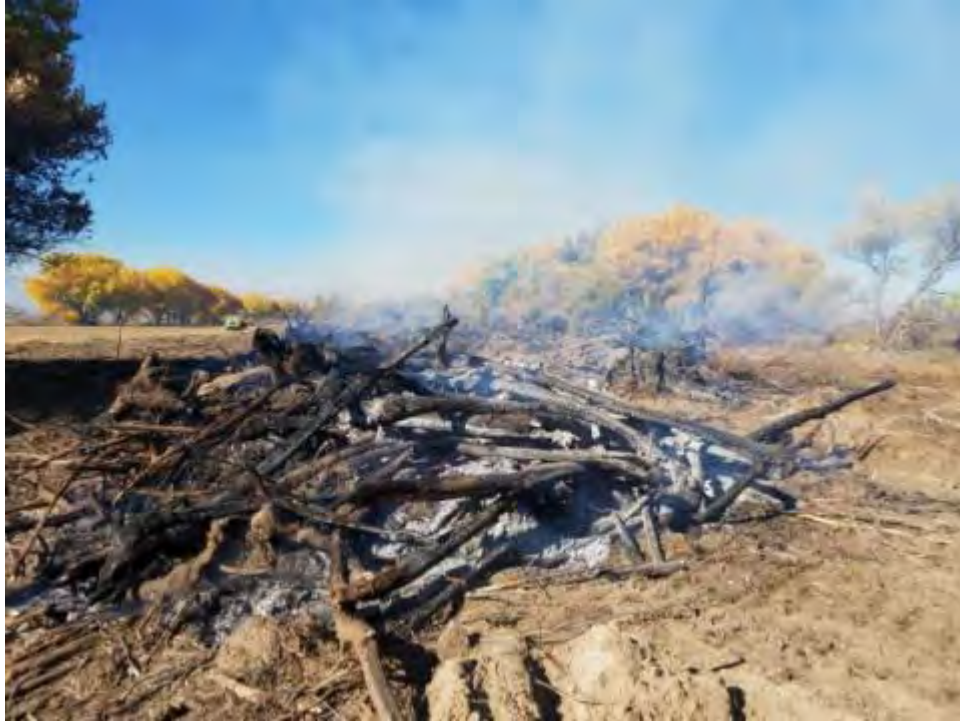
Salt cedar piles being burned. The water pumper truck can be seen in the background.
