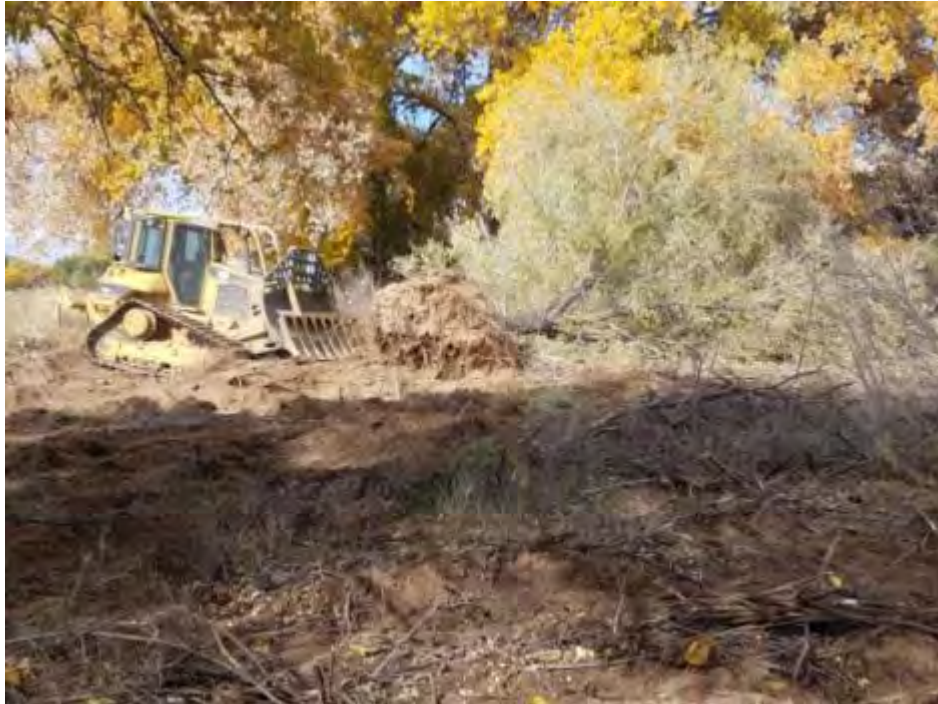
Contractor pushing above ground brush over to prior to root plowing/raking.
