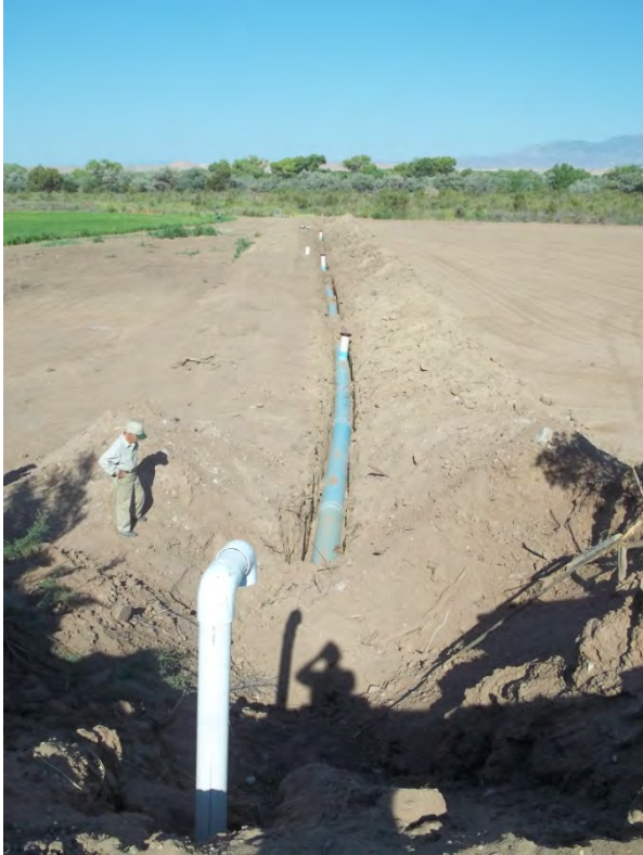
JMC Farms Irrigation Pipeline installation
