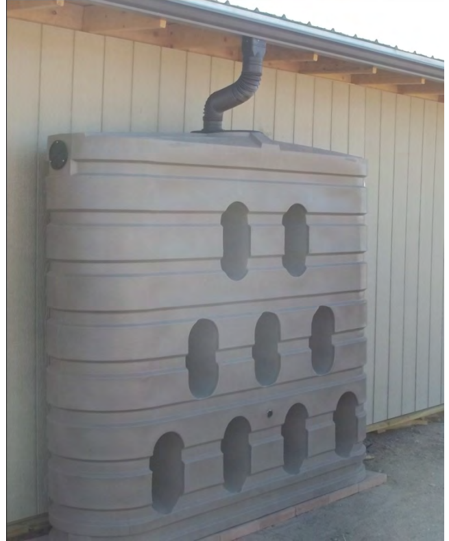
Installed rain barrel system
