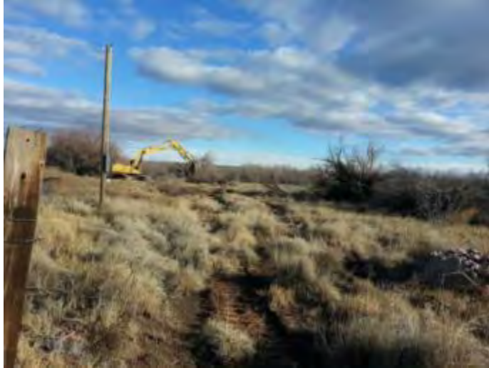
The excavator begins work, January 2015
