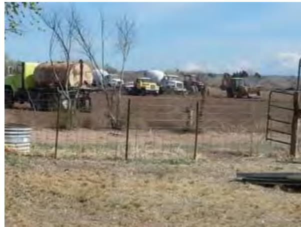
Tractors pulling boat and concrete trucks delivering concrete into boat as ditch is poured.
