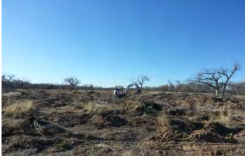
A small area following excavation at the Socorro Nature Area.
