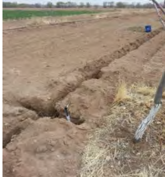
SWCD cooperater installing underground drip.
