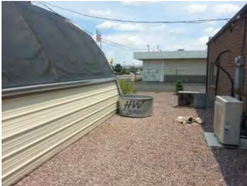
South side of greenhouse. Gutter is just below the black shade cloth covering the greenhouse. Gutter pours into large round stock tank that is hooked to stock tanks inside greenhouse.
