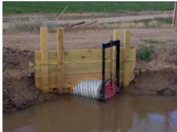
Turnout replacement, Lemitar, NM.
