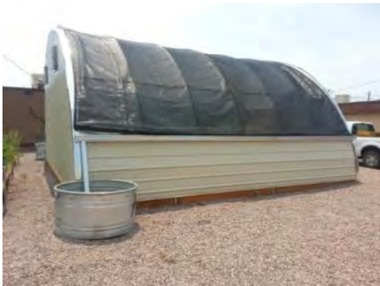
North side of greenhouse. Gutter and stock tank to collect rainwater on this side also.
