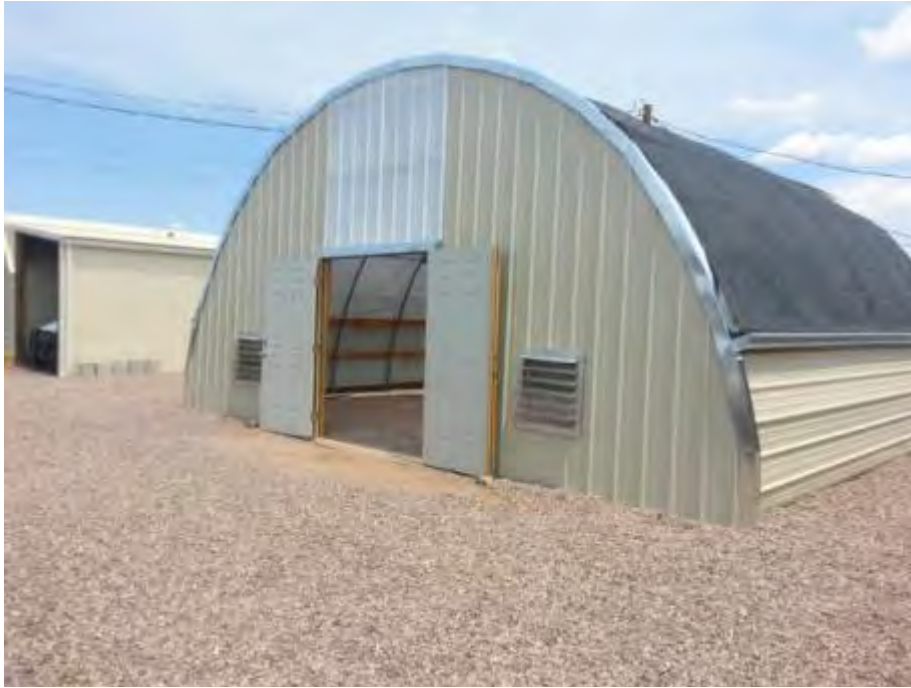
West side of greenhouse. Aluminum shutters open every morning once the temperature goes above 70 degrees F. French doors allow access to inside of the greenhouse.
