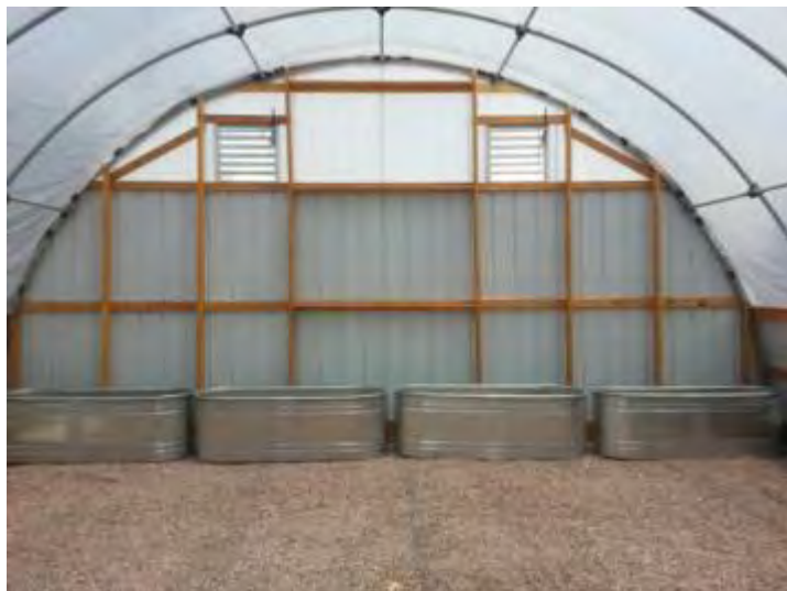
Inside of greenhouse (east wall). Stock tanks that will hold water to run micro-sprinklers.
