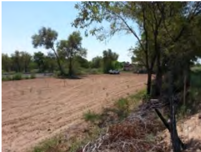
Land leveling in Sabinal, NM.
