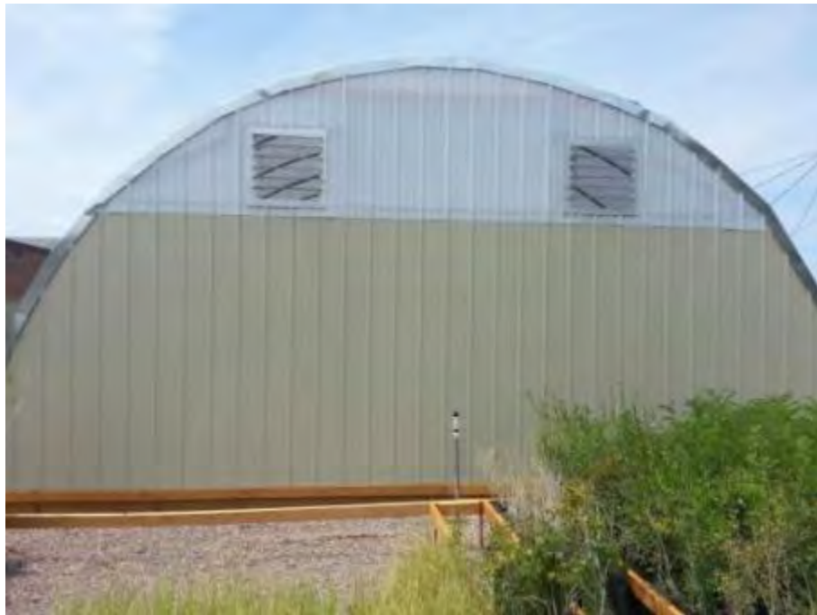
West side of greenhouse. Aluminum shutters are elevated on this side of the greenhouse.
