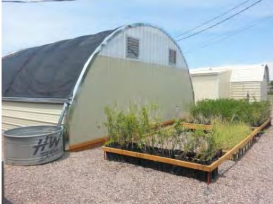
East side of greenhouse. Current plant stock in outside shrub cages, where they are watered each morning.
