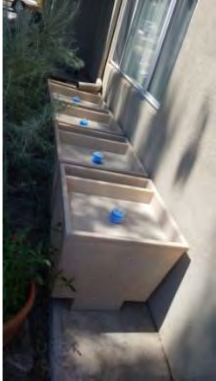
Set of four connected rain barrels. This type allows you to plant on the top of the rain barrel and moisture wicks up to the plant roots.
