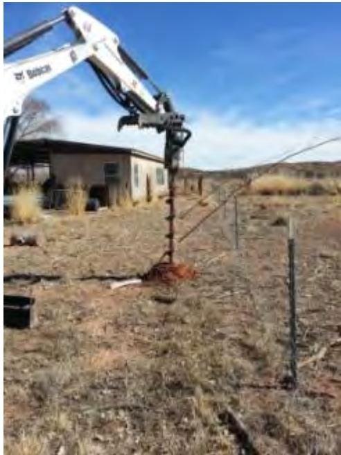
Using the Bobcat to auger holes-Saavedra.
