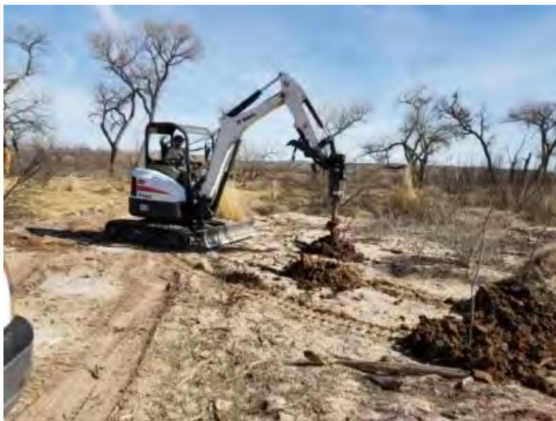
Drilling holes for the Gooding's willow poles to be planted in.
