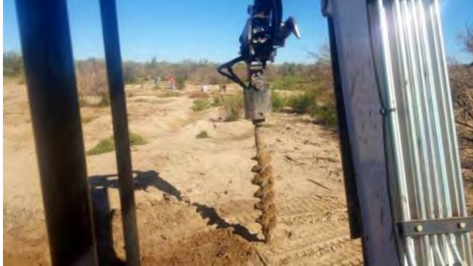
Bobcat and auger used for drilling holes for planting.
