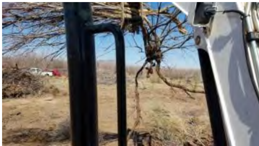
Extracting and piling salt cedar on the Rhodes-adjacent BLM property
