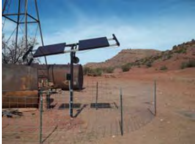
Solar panel conversion, livestock well, Bingham, NM.
