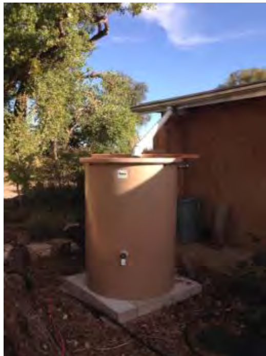
Rain barrel collection system in Socorro, NM
