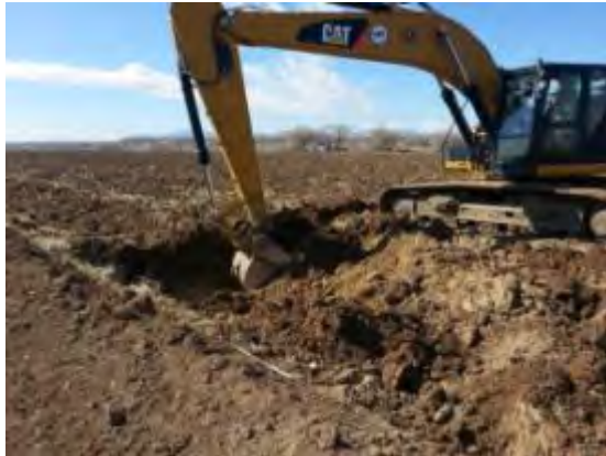
Sub-soiling in San Antonio, NM.
