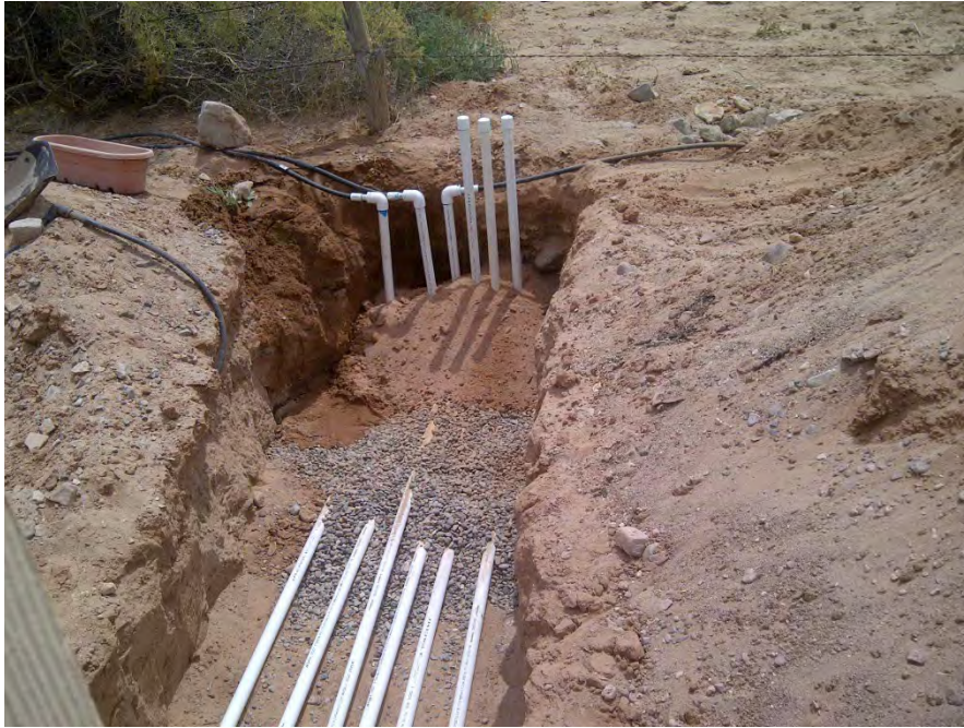
Installation of a six-zone drip irrigation system.
