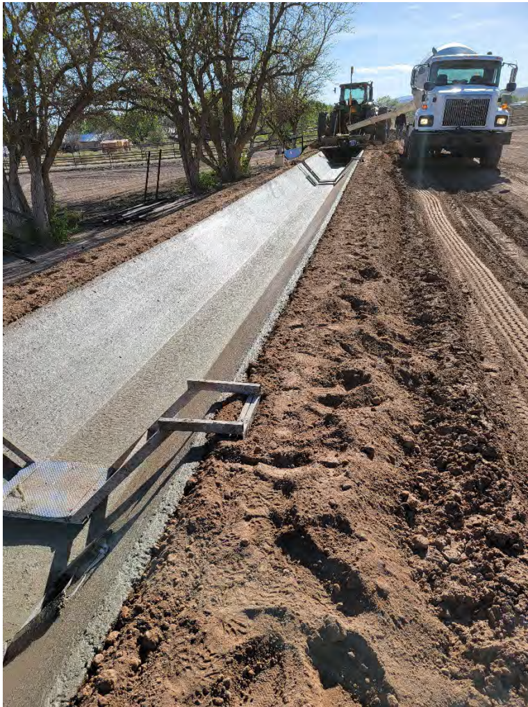
CTA provided to a local farmer installing concrete ditch.
