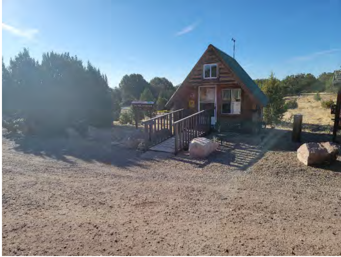
Above - Datil Well Campground entrance area.
